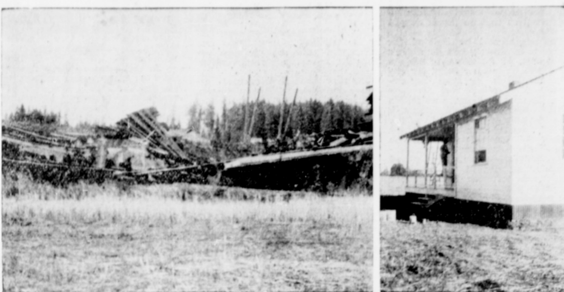
These pictures tell an interesting story of rural rehabilitation work in Washington county. On the left is a broken-down building, worn by the ravages of the winter storms. On the right is a home of the type being erected under the federal program—white, neat and spacious enough to handle the needs of almost any farmer. The rural rehabilitation program is providing several such "resurrections" for Washington county farmers, turning back to them the refurbished property.
