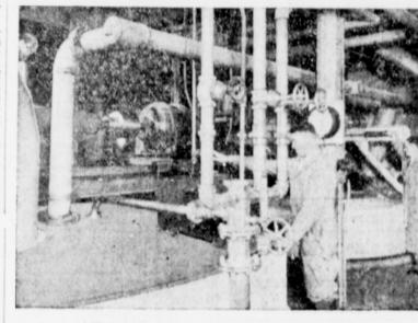
Mash cooker and mash strainer, showing mashing process temperature control.
