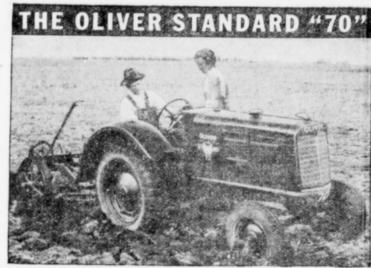
When you own an OLIVER 6-cylinder "70" you have a right to be proud because it is the most modern tractor money can buy. Fast, easy - handling, easy - riding—more work done with less fuel used. Pick a motor for the fuel you prefer. The "70" High Compression for regular gasoline. The "70" KD for kerosene or distillate. Each designed for maximum fuel economy.
