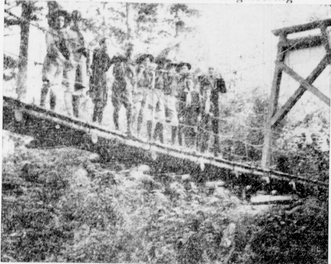
When friends, and sponsoring organizations of Boy Scout troops in the Hillsboro district, attended the dedication of Camp Elizabeth Ireland Thursday night, access to the camp was by way of a 100-foot suspension bridge across McKay creek. The bridge, shown above, was constructed by scouts under the direction of Scoutmaster Tom Bronleewe and his son. The bridge is deemed an excellent piece of engineering—Cut courtesy of The Oregonian.
