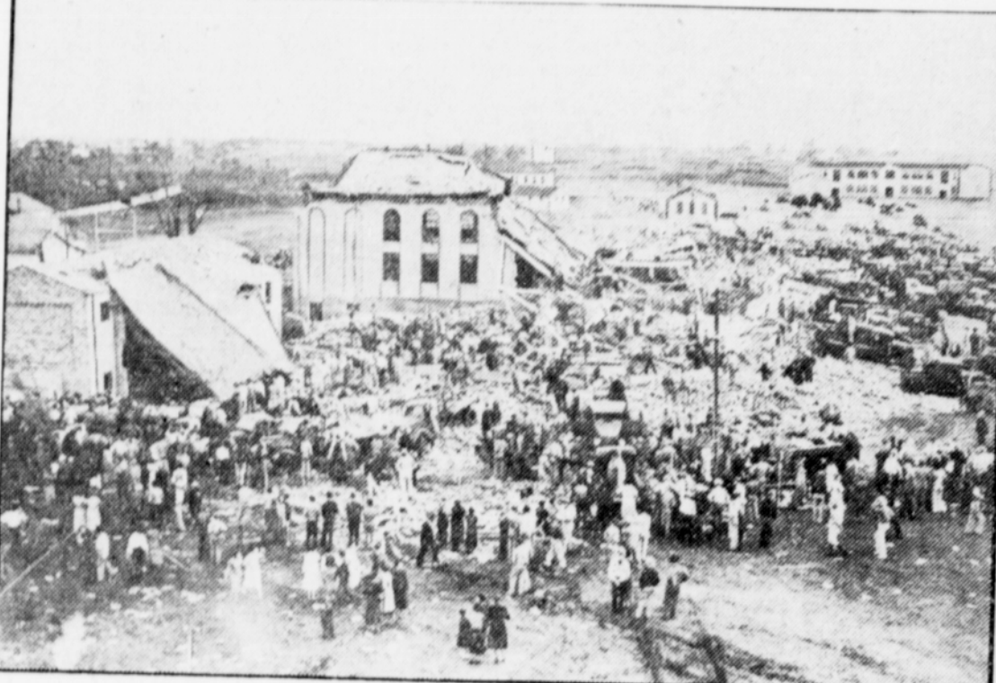
A terrific gas explosion, 10 minutes before dismissal time, left this scene of grim disaster at the New London, Texas, consolidated school. At least 425 students and teachers were killed and 125 injured when gas, accumulating in the school's basement, suddenly ignited and shattered the two-story structure into a mass of tangled wreckage. Bricks and timber and debris were hurled hundreds of feet. The force of the explosion was felt three miles away. Children were horribly mangled. More than 1000 students were in the building at the time. One of the richest schools in the world, it is situated in the heart of the East Texas oil fields, and has 11 wells on its own grounds.
