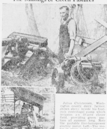
tor in place under a protect-ing roof. Illustrated courtesy Portland General Electric
