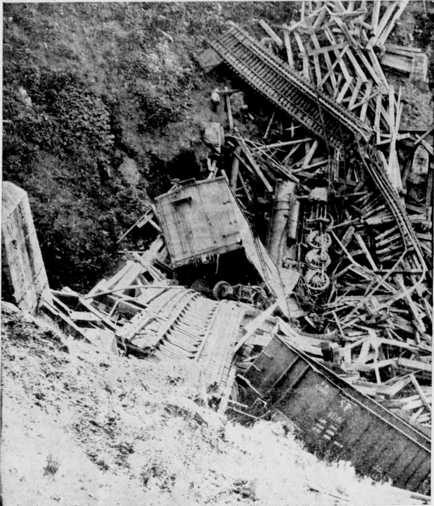
Five men went to their death August 6 three miles west of Cochran, Washington county, on the Southern Pacific Tillamook branch when a wooden trestle gave way under the Tillamook bound freight train. General view, taken from the side from which the train rode onto the trestle, spanning Little Baldwin creek, shows remains of the broken trestle piled amid the engine, box car and gondola that went over. The rest of the 38-car train was stopped. Engineer, fireman, two brakemen and one bridge worker met death in the crash, one of the most disastrous in the history of the Southern Pacific.
