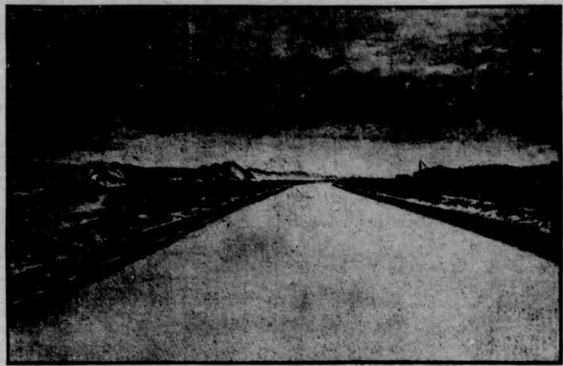
CANAL AS SEEN AT WILLOW SPRINGS—LOOKING WEST.
