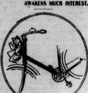
The Bettis "wind motor" may be de scribed as the paramount curiosity of the Stanley bleyele show in England. It consists of a rotating fan, set in motion on meeting a wind, and two sets of beveled gearing at the ends of a revolving shaft. The spindle of the fan is attached to the upper pair of cogs, which turn the shaft. This operates the second pair, which are in front of the crank bracket, and they in turn engage with a toothed wheel which sets the crank axle in motion.
