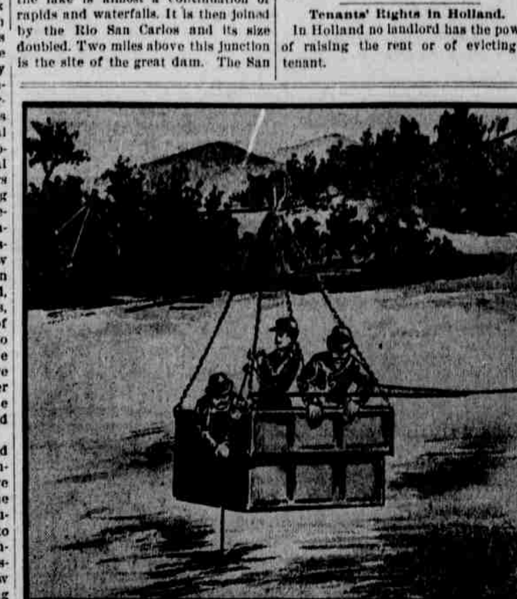
NICARAGUAN ENGINEERS FINDING RIVER LEVELS.
