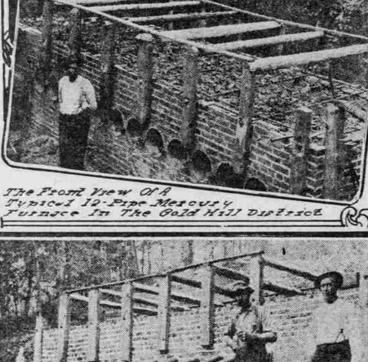
The Front View of a Typical 10-Pipe Mercury Furnace in the Gold Hill District
