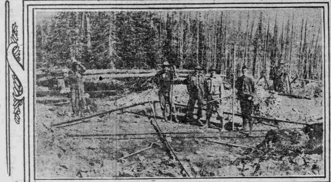
Building Dike For Mill Tower On Summit Of Wenatchee Range
