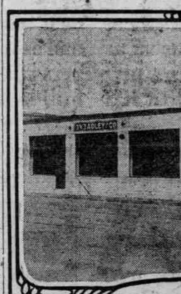
Structure at 440 East Morrison street just completed and taken over by tractor distributing firm.
