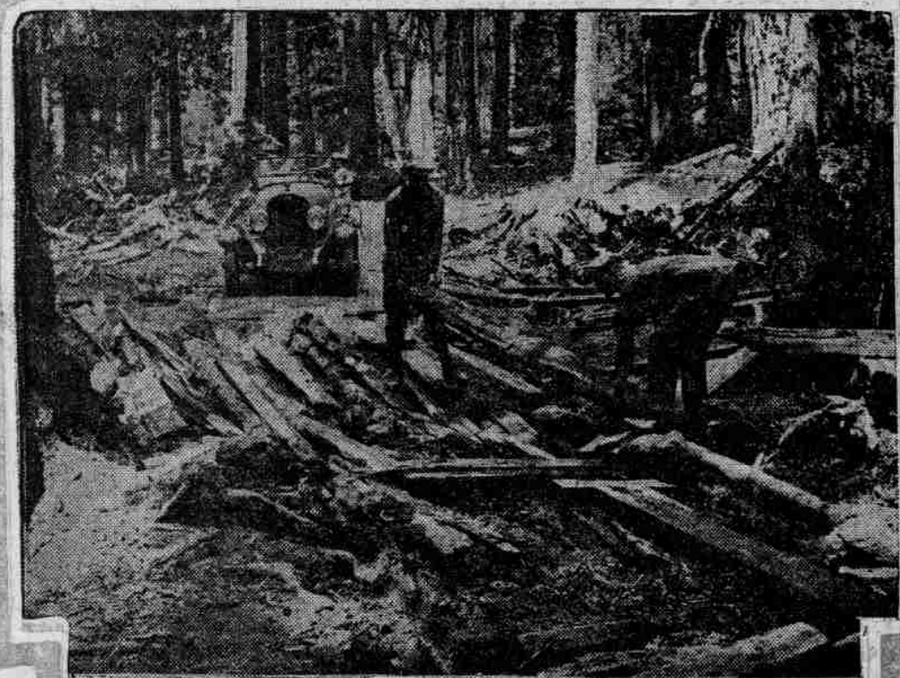
Bridging a swamp was part of the day's work
