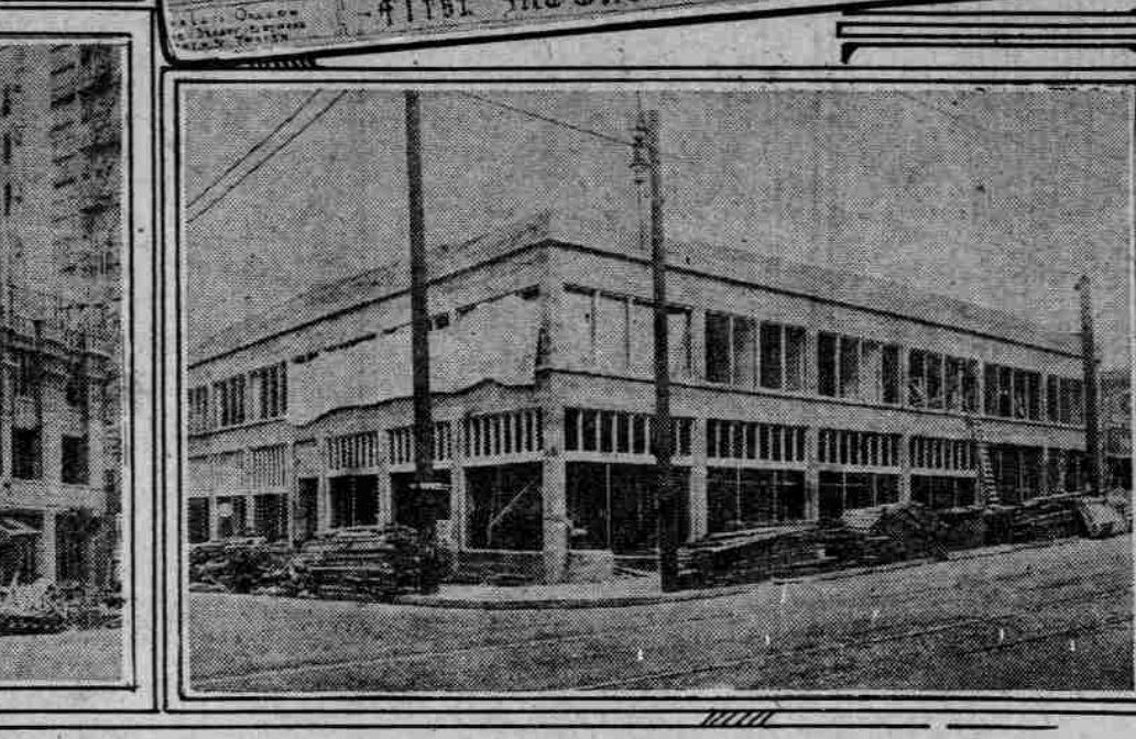
Above at left—New residence of Lloyd R. Smith in Georgian Court district. Above at right—Sketch of proposed $100,000 First Methodist Episcopal church at Corvallis, by DeYoung & Rosdahl, architects. Below at left—$100,000 storage garage building now being erected for Imperial Investment company at Fourth and Pine streets. Below at right—Building to cost $35,000 being erected for Boyer Printing company at Tenth and Yamhill streets.
