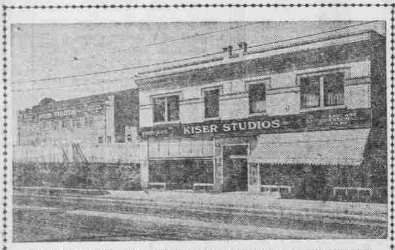
"CLOSE-UP" OF THE RECENTLY COMPLETED AND FINELY EQUIPPED STUDIOS OF FRED H. KISER IN THIS CITY.
