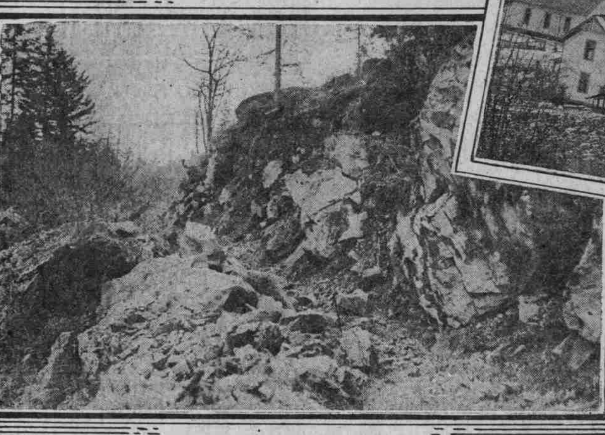
Rock Cut Ready for Rails.
