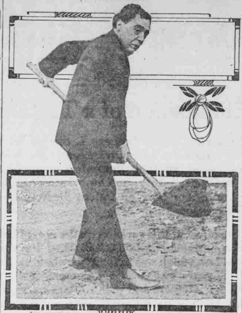
D. Solis Cohen, who lifted first earth with golden shovel at Eleventh and Alder streets last night.
