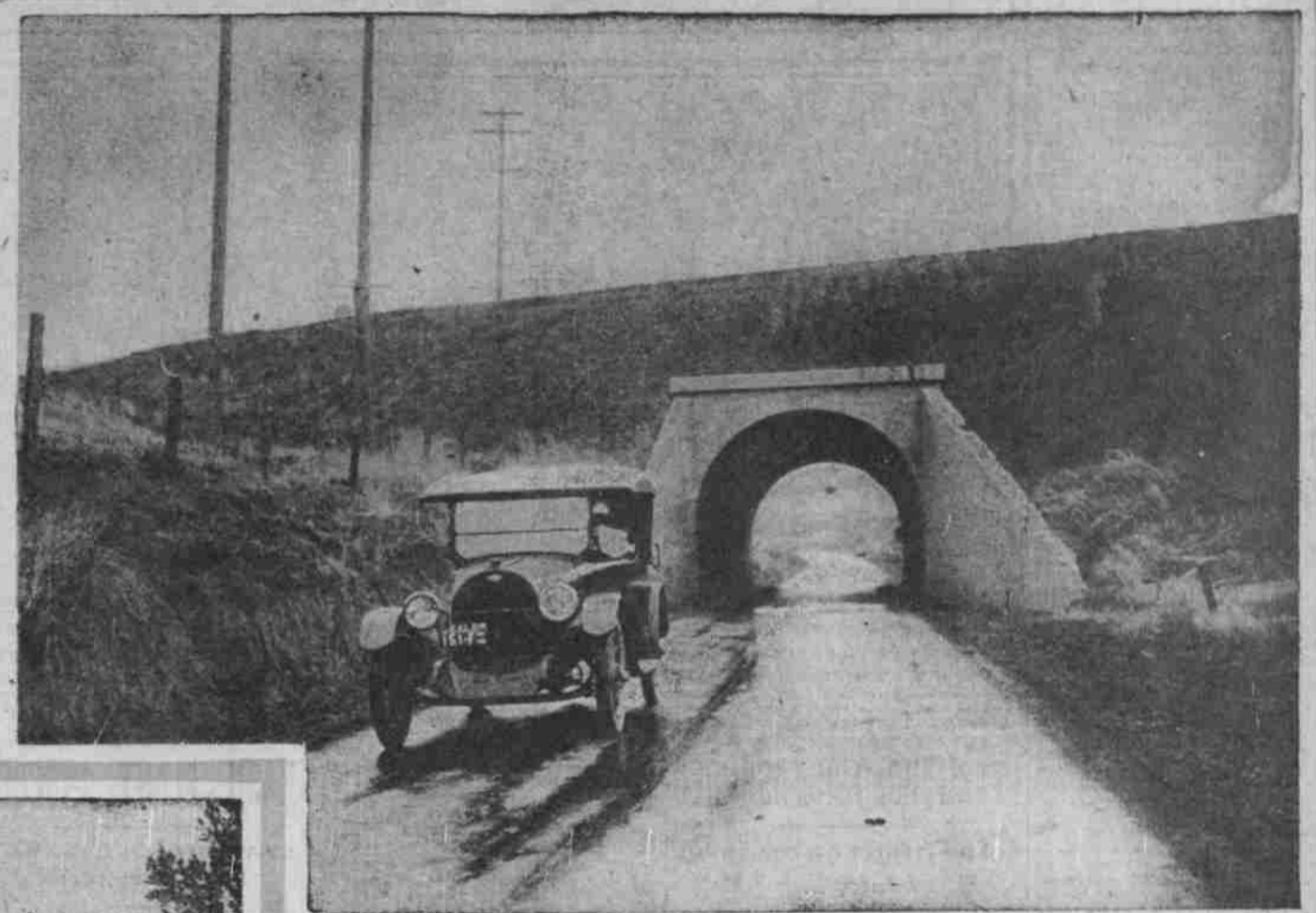
Chevrolet Car at Tunnel Under Railroad Near Pendleton.
