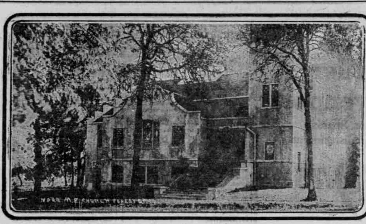
First Methodist Episcopal church of Forest Grove, where sessions of the annual Oregon conference of the Methodist Episcopal church will be held, starting October 5.
