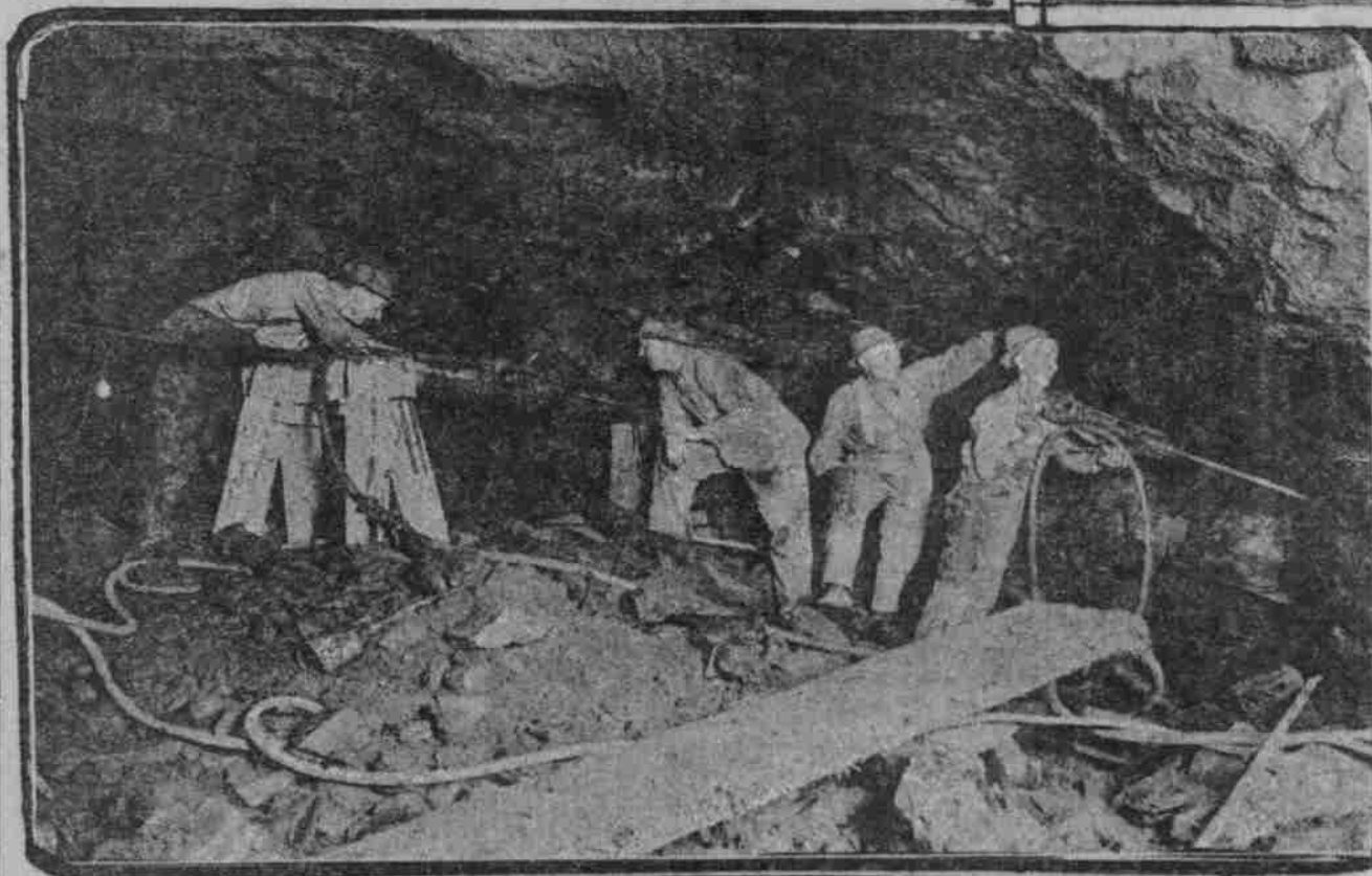
Pneumatic Drills on Top Bench of Tunnel Heading.
