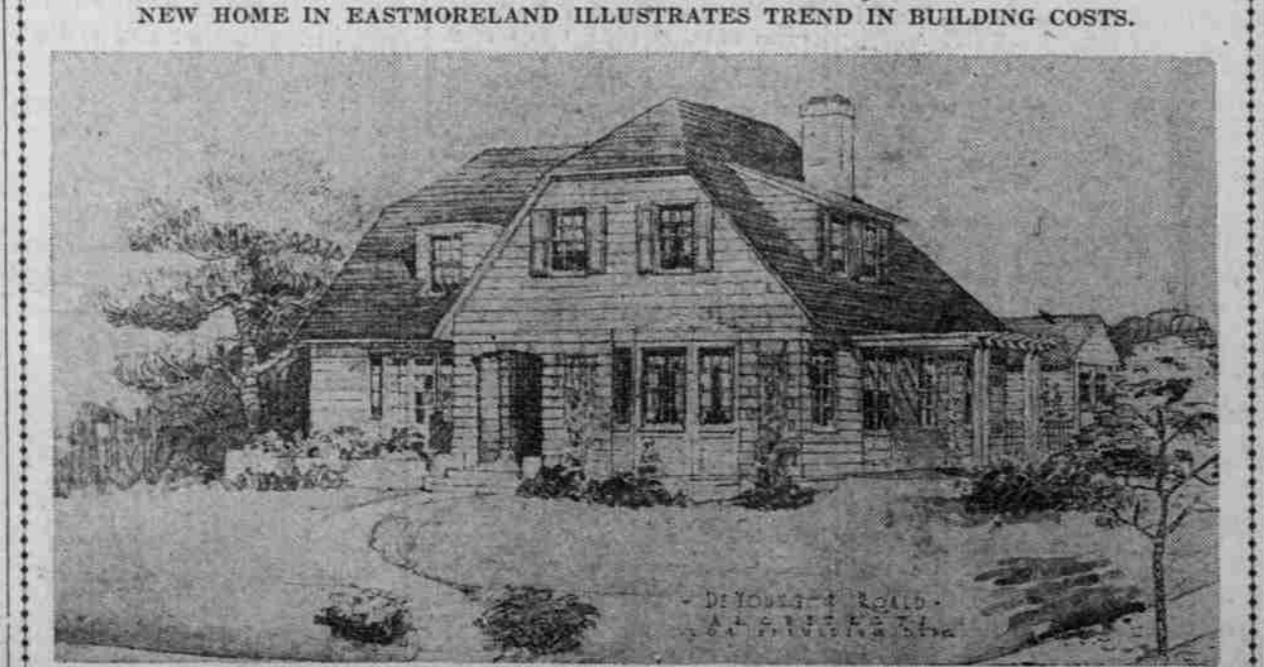
STRUCTURE IS BEING ERRECTED FOR R. C. DIEBENKORN AT $3000 SAVING.
