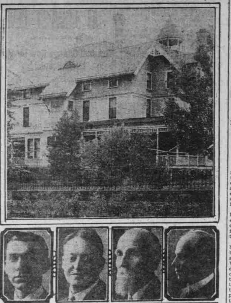
Top—Residence altered into church edifice. Below, left to right—R. B. Cox, A. F. Jack and L. P. Horton of building committee and Rev. Melville T. Wire, pastor.
