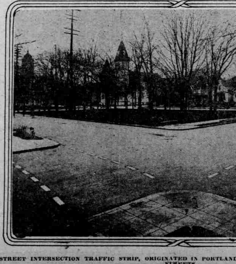
STREET INTERSECTION TRAFFIC STRIP, ORIGINATED IN PORTLAND, LAID AT WEST PARK AND CLAY STREETS.
