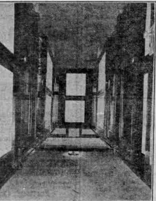
Showing Hallway With Rest Rooms on Each Side, Equipped With Regular Hospital Beds.
