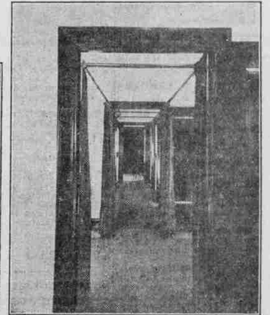
Long Hallway With Treating Offices on Each Side.
