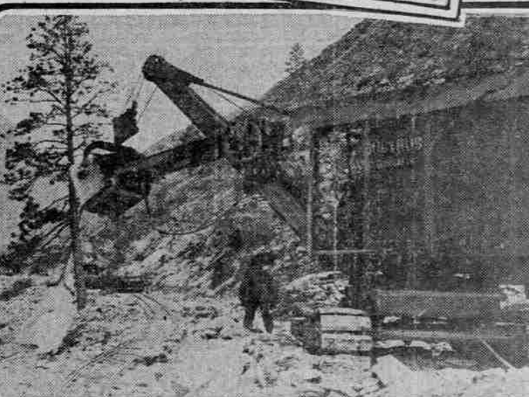
The Big Steam Shovel at Work in the Salmon Canyon.
