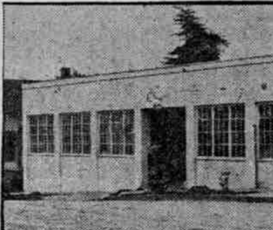
CONCRETE STRUCTURE AT EAST SEVENTH AND UMATILLA AVENUE IS WELL EQUIPPED.
