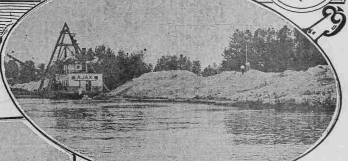
This High Dike Will Curb Flood Waters.
