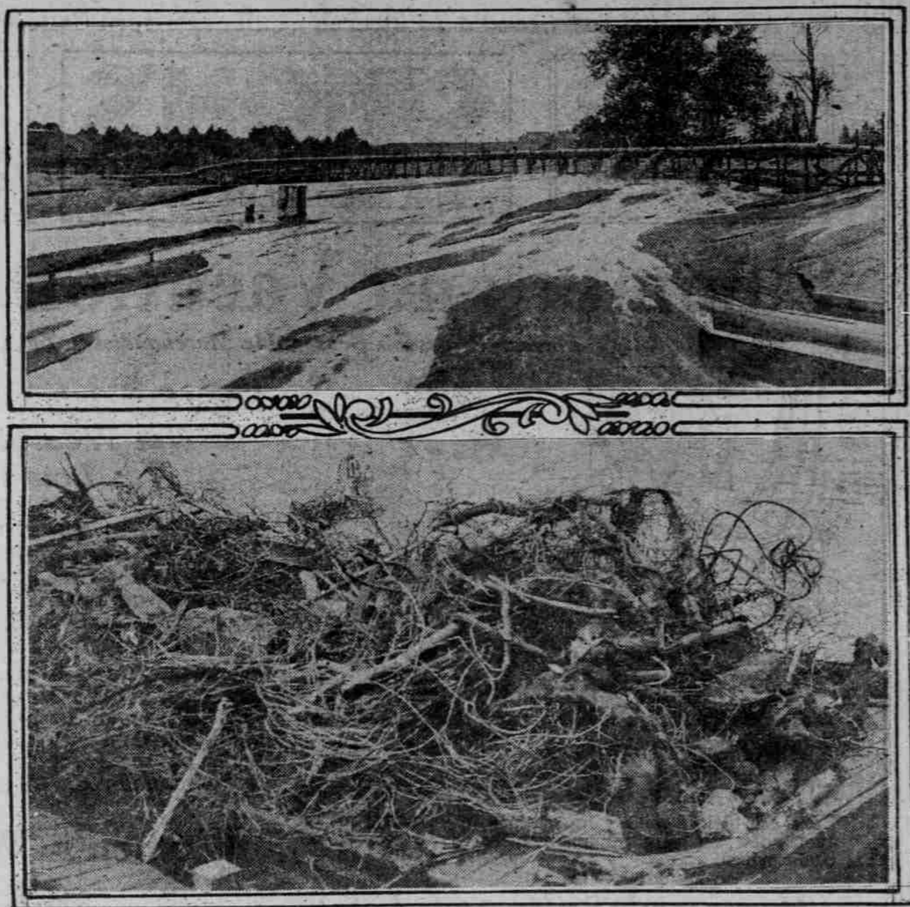
Above—Dredge Portland filling site for bunkers at municipal terminal No. 4. A spectacular bit of dredging was done here in raising the material from the river bottom to an elevation of 44 feet above water and depositing it through a stotted pipeline.
