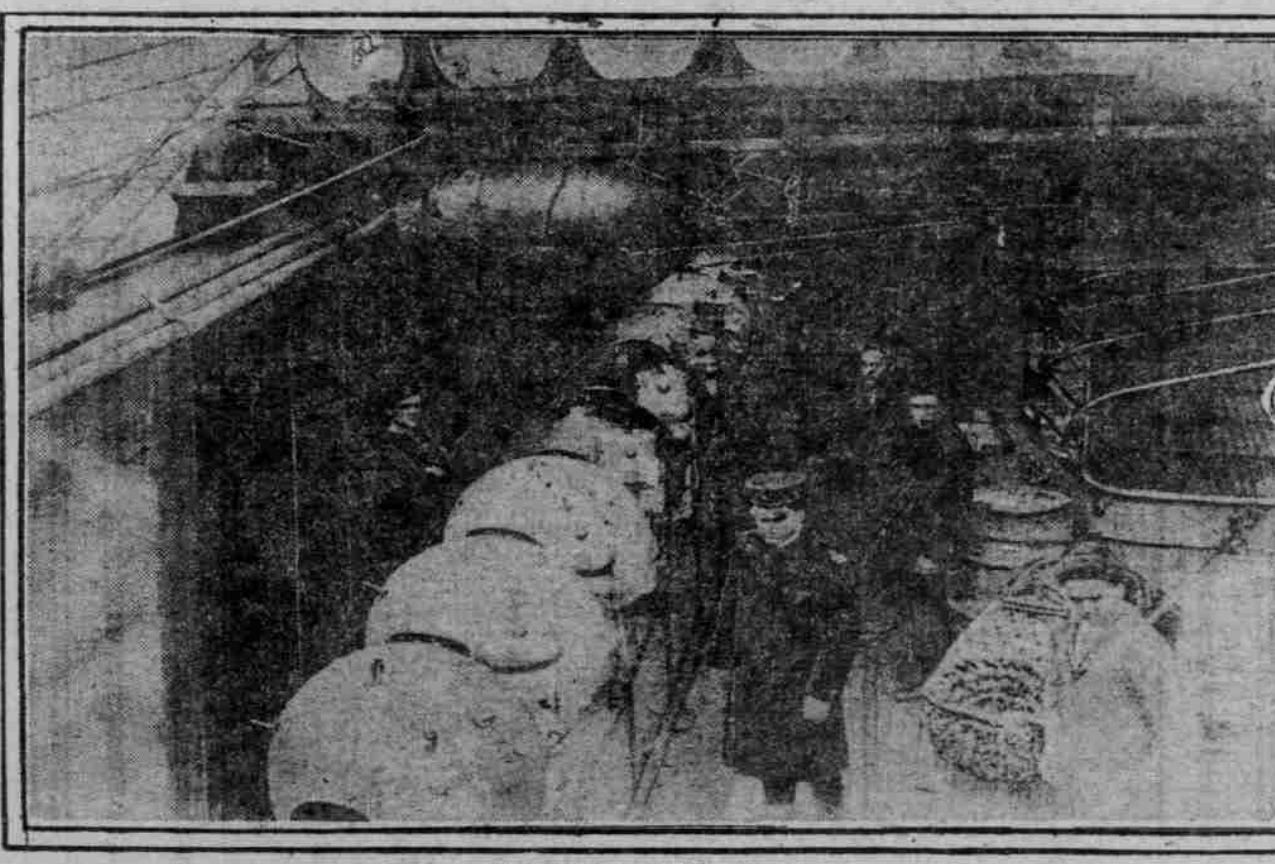
ON THE LAUNCHING DECK. The mines moved on little railroad tracks toward the stern, whence they dropped, at about ten-second intervals, into the water. Each mine-laying ship carried about 500 on an average.
