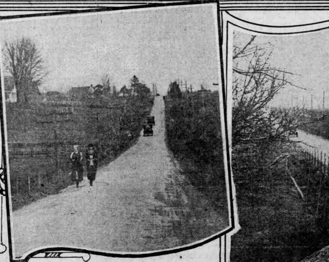
HERE are some views along the new paved highway to Beaverton, Reedville, Hillsboro, Cornelius and Forest Grove. The pavement has been extended from Hillsboro to Forest Grove only within the past few weeks. This highway, which cuts through the rich Tualatin valley, was opened to Beaverton and Hillsboro only a couple of months ago, but already the paved turnpike is crowded with cars on Sundays. The road is one of the straightest in the state, there being not more than half a dozen main curves all the way from Bertha station, just outside Portland, where it branches off the Capital highway, clear to Forest Grove. Above at the left is one of the few curves in the highway, this being near Reedville. At right—Big oil tanks of Union Oil company of California, at Cornelius. Center, left—Pacific university at
