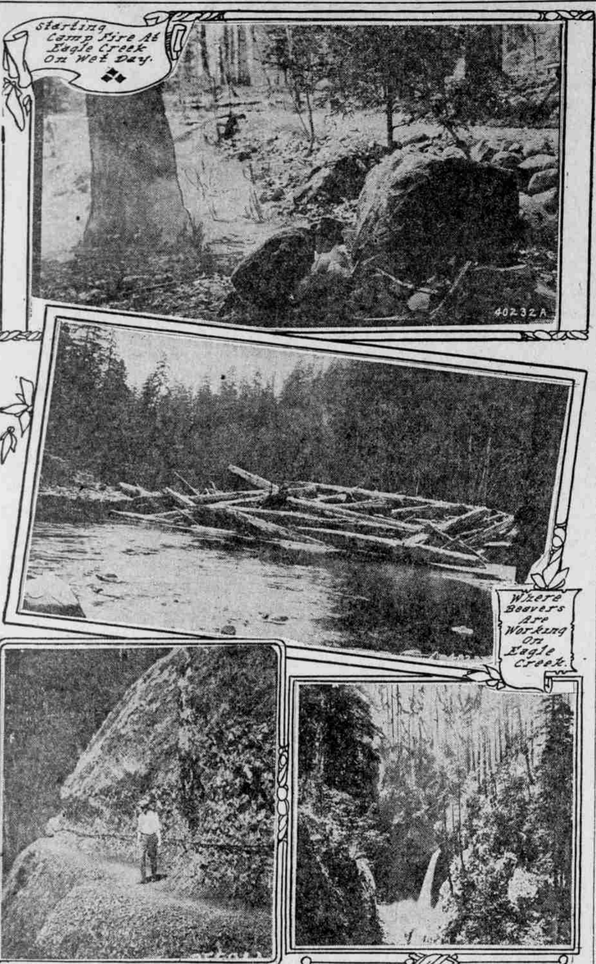
Rock Cut on Eagle Creek Trail. Metlako Falls.
