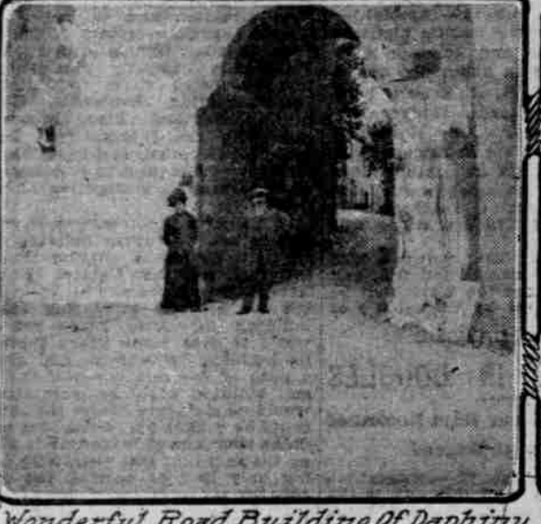
Wonderful Road Building of Dauphine In France.
