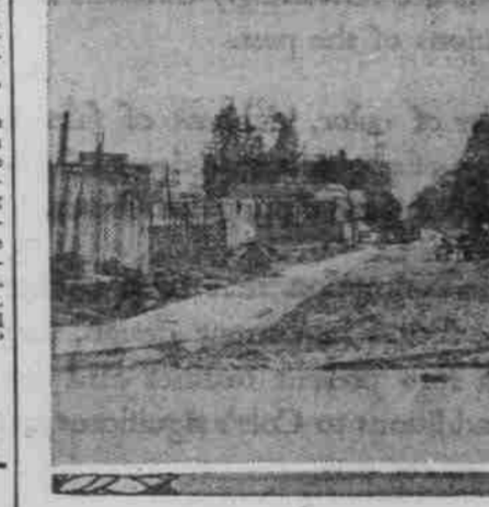
Morrison street between Nineteenth and Twentieth at last to be paved. The city took the contract for hard-surfacing it and, as shown in the picture, rock is being spread preparatory to applying the "hot stuff." Its completion should relieve some of the traffic congestion at Nineteenth and Washington by providing an outlet from Nineteenth on Morrison straight through to upper Washington.
