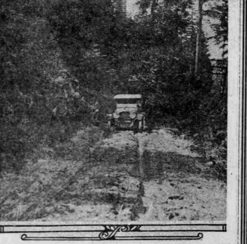
This picture was taken near the summit of the long climb over a ridge which the old road takes between the gravel pit beyond Herman Lake ranger station and Wyeth. This detour is 3.6 miles long. In wet weather it is soft and bad.
