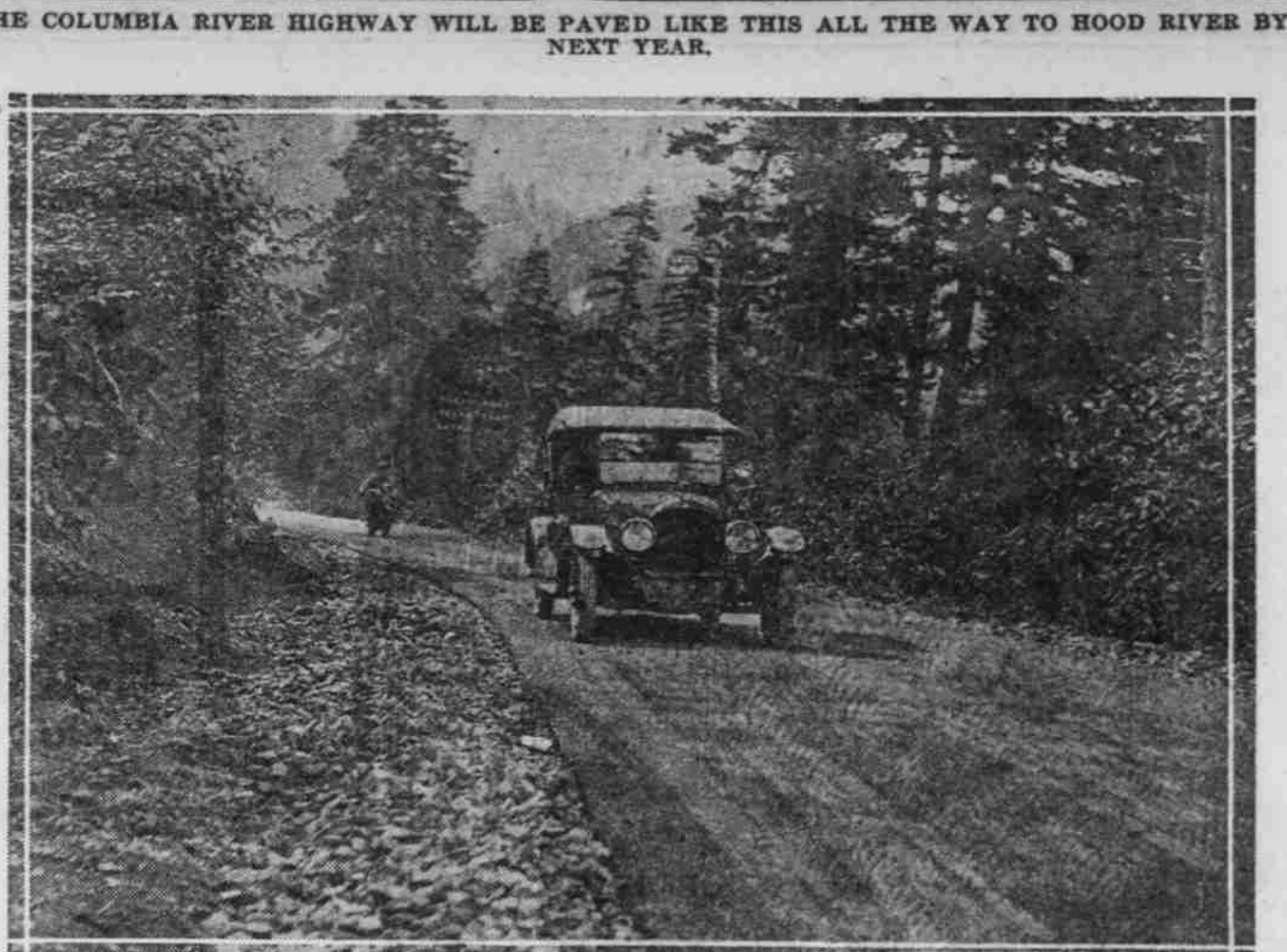
This picture shows a section of the newly complete bitulthle pavement between the Multnomah county line and Cascade Locks. A mile and a half more of this particular stretch remains to be paved. Cars can go through only before 7 o'clock A. M. and after 5:30 o'clock P. M. while this construction is in progress. The car in the photo is a Willys-Knight.
