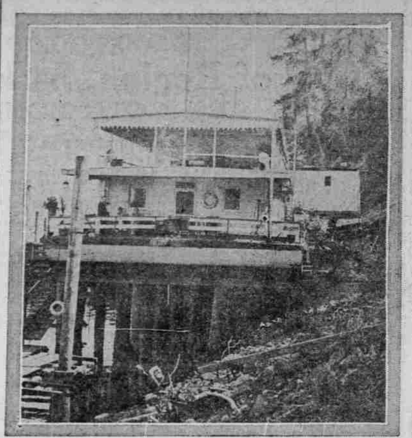
HOUSEBOAT ELVIRA, OWNED BY J. J. MCCARTHY AND L. A. WEST, UNDERGOING REPAIRS IN ITS HOME MADE DRYDOCK AT RIVERDALE.
