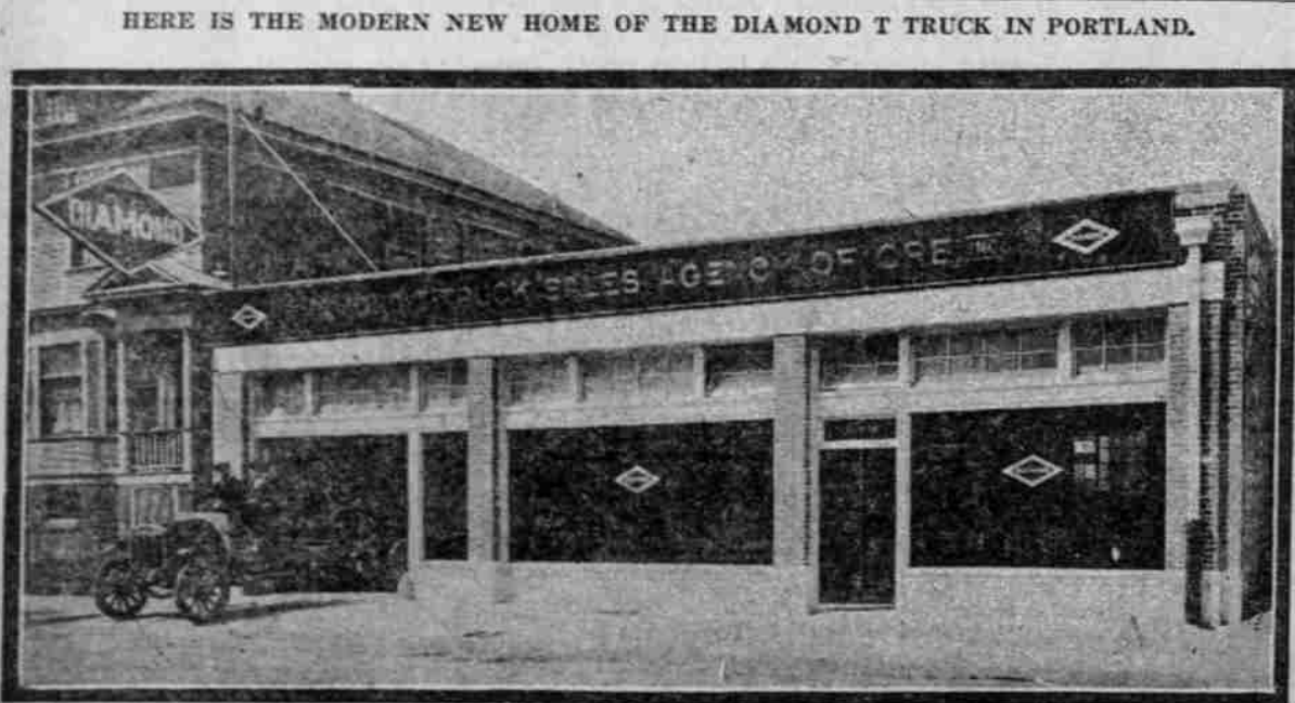
New building just occupied at 80-91 North Ninth street, near Flanders, by the Diamond T Truck Sales Agency of Oregon. August Jung is president of the company, and as Diamond T distributor has placed a great number of these trucks in Oregon in the few months since he took the agency here. The building was erected especially for him on a five-year lease to provide imperatively needed larger quarters.
