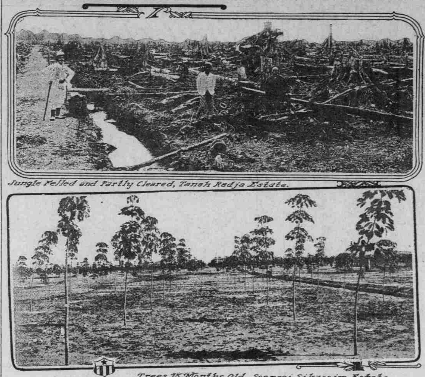
Jungle Felled and Partly Cleared, Tanah Radja Estate.
