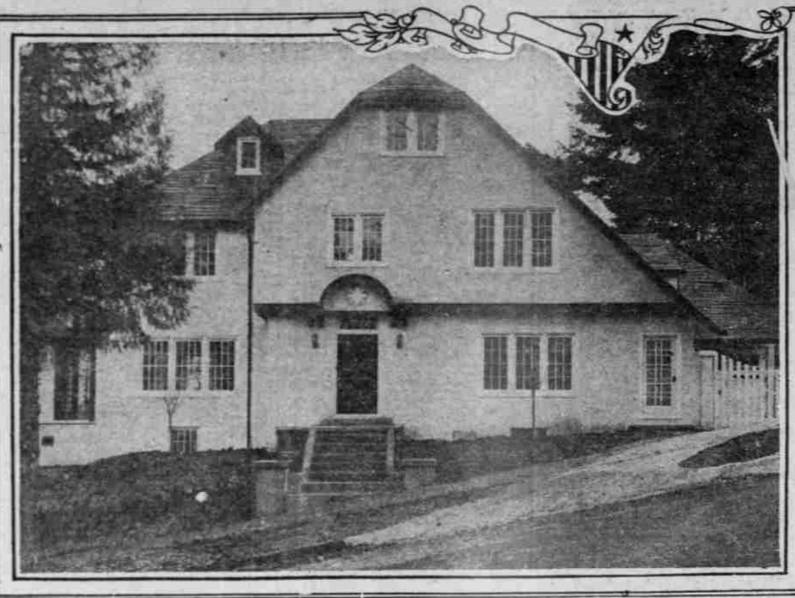
MODERN RESIDENCE CONSTRUCTED BY F. E. BOWMAN & CO. AT COST OF $12,500.
