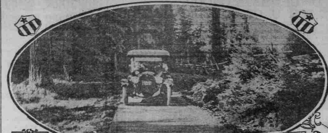
Stretch of New Plank on Mt. Hood Road, Near Aschoff's.
