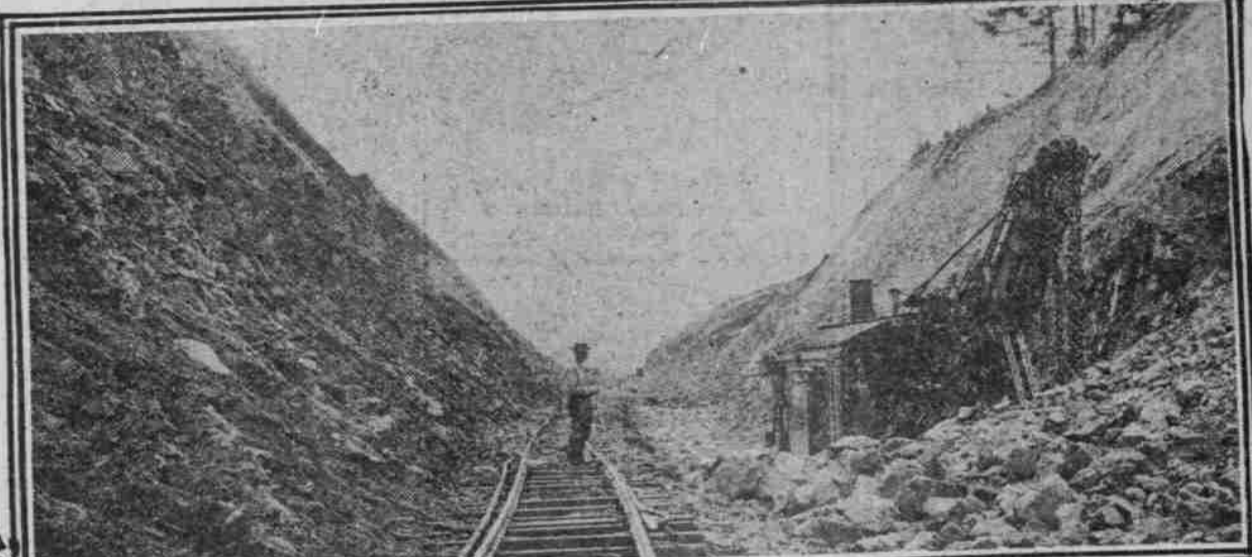
Steam Shovel Making 60ft. Cut. Arthur Porter, Contractor In Foreground.
