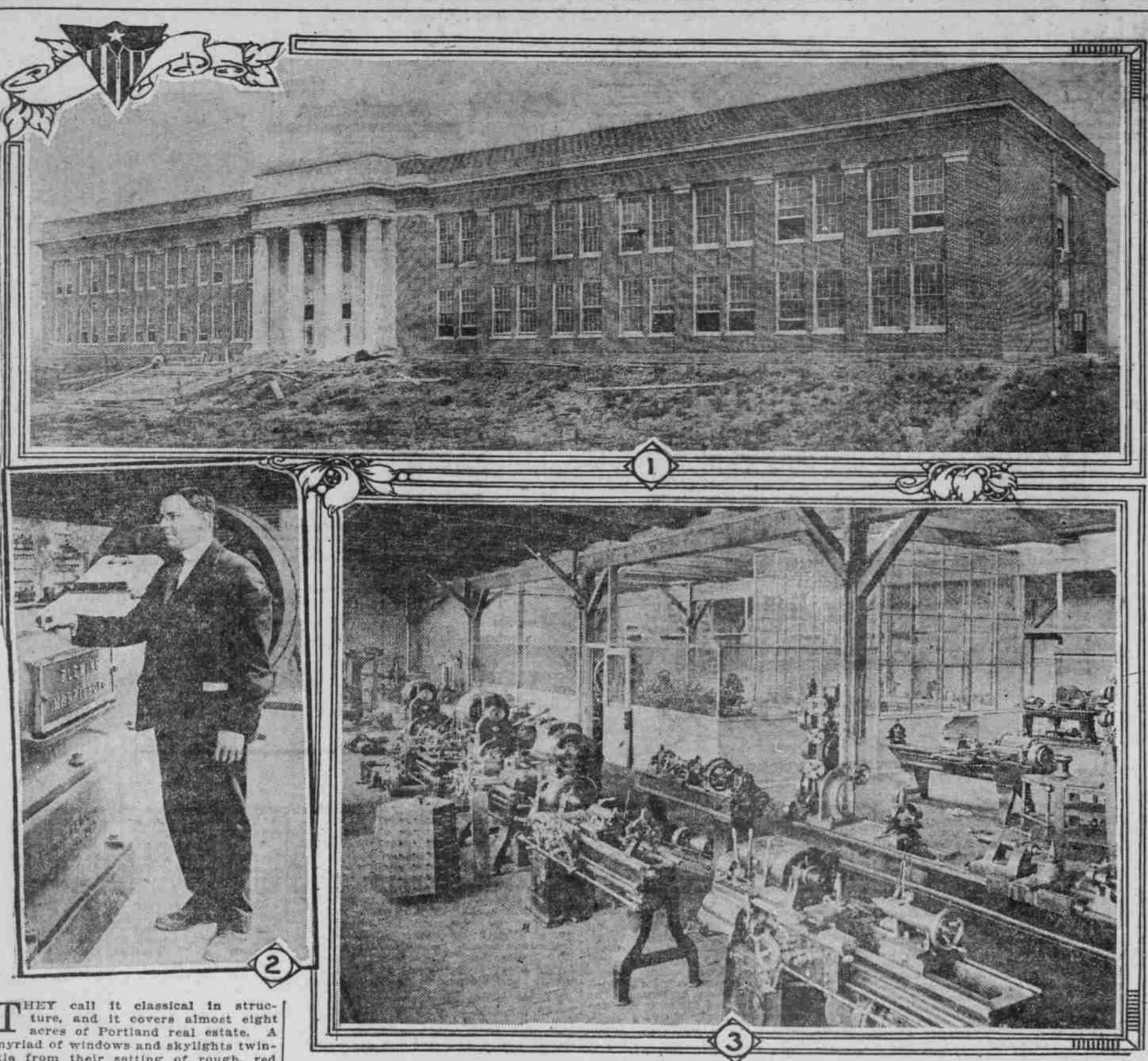
1—Administration Building and Main Entrance, Facing West on East Twelfth Street. 2—C. E. Cleveland, Principal of the Benson, Admiring the School's 300-Horsepower Engine. 3—Partial View of the Great Machine Shop, With Battery of Lathes in Foreground.
