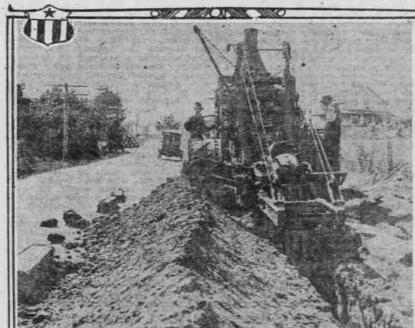
OVA Trench Digger Capable of Digging a Ditch Seven Feet Deep and Twenty Feet Wide
