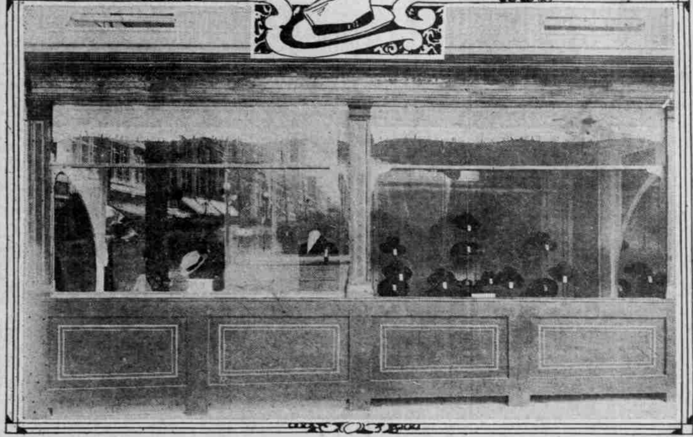
At Left Is the Temporary Straight Window Glass Which Mirrors Street Scenes, While at the Right is the New Concave Glass Window in the C. J. Mathis Company Store, Corbett Building, Which Eliminates All Reflections.
