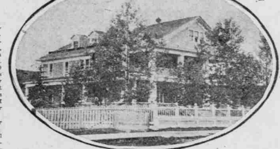
The Commissioner's Residence.
