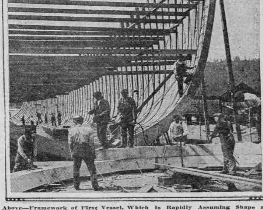
Above—Framework of First Vessel, Which is Rapidly Assuming Shape at the Yards. Below—End View of Same Structure.
