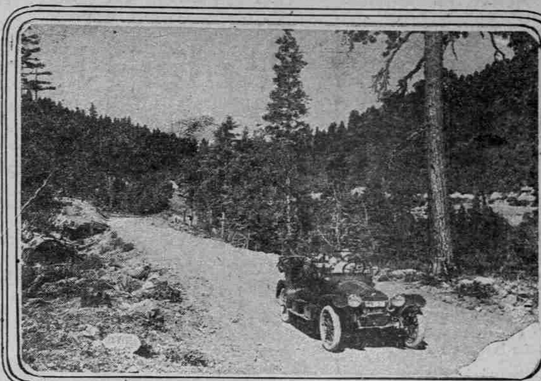
New Highway Over the Siskiyou Mts. Near Oregon-California Line
