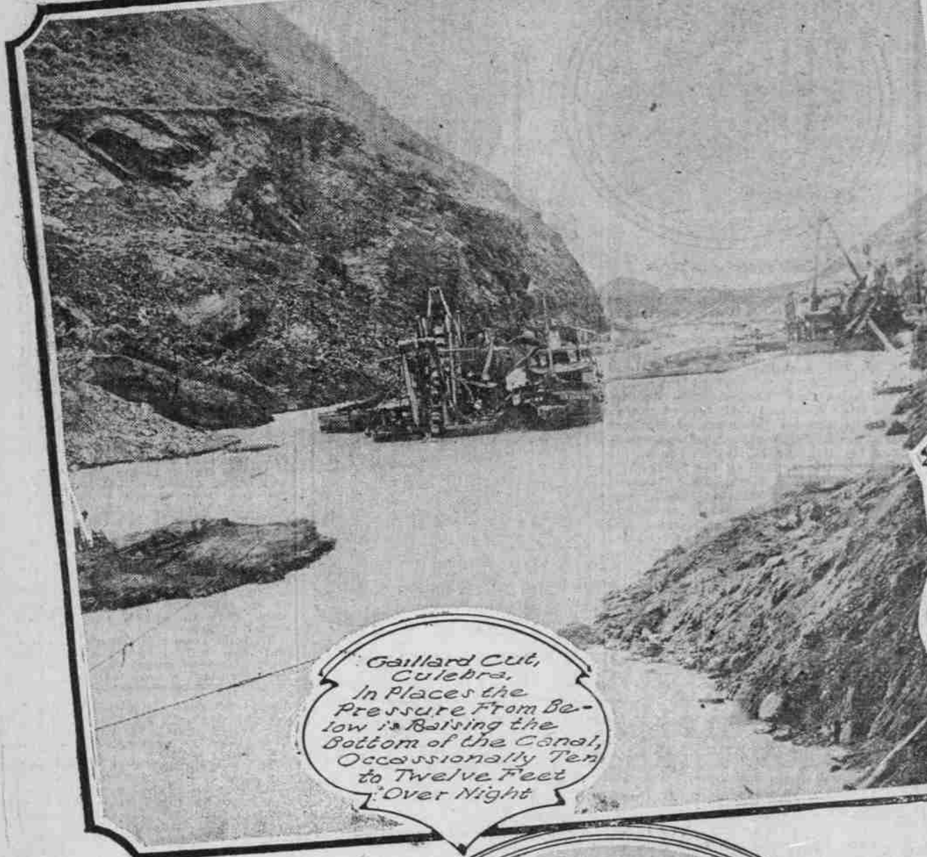
Gaillard Cut, Culebra, Looking North From Contractor's Hill, Showing Barrier Across the Canal. This Picture Suggests Subterranean Dis- turbance in and Across the Canal.
