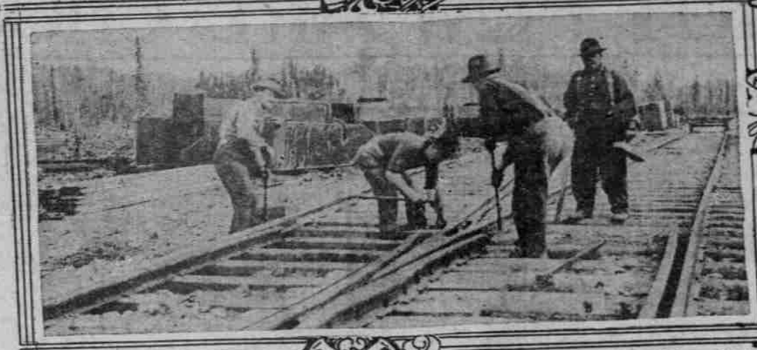
Laying the Tracks.
